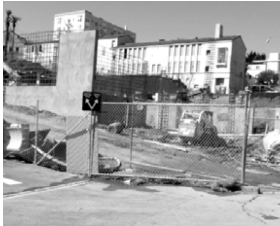
Construction site at 55 Laguna
